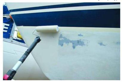
**Eroding antifoulings** use the water's friction to reduce the thickness of the paint and expose fresh layers of biocide. This erosion releases biocides in a controlled manner, providing a longer and more consistent performance throughout the season. It also helps to reduce long-term build-up of antifouling.
