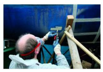
**PBO VERDICT:** A slow but easy way to remove antifouling. You could save money by grouping together with fellow boat owners to share a blasting unit. Hiring a large compressor (30-40cfm) would make the job much quicker.
